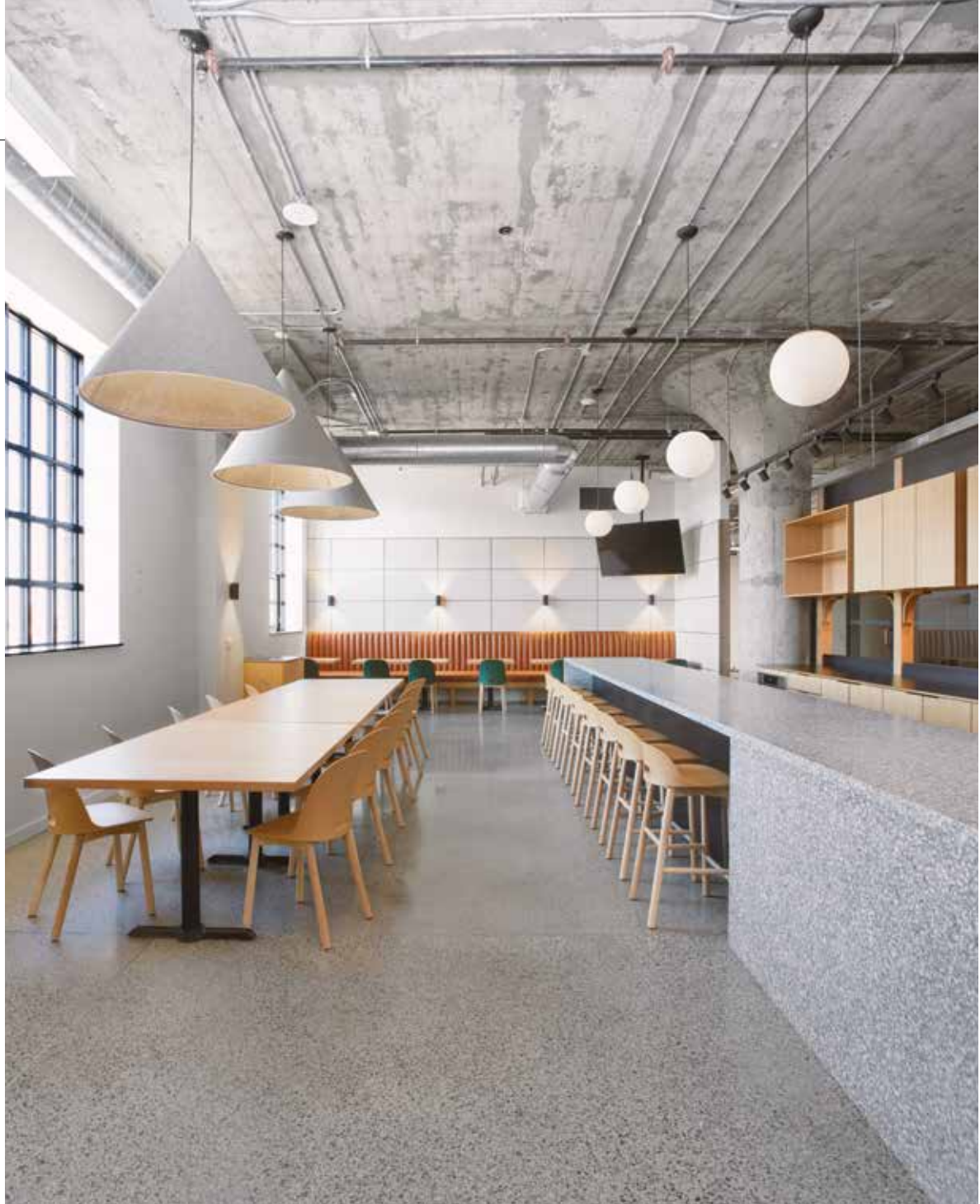
→ The kitchen's terrazzo concrete bar was cast to match the original factory floors
